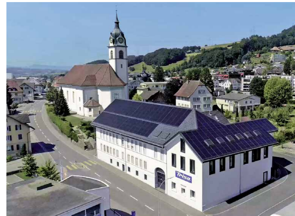
▲ On the flat roof of «Werk 2», a state-of-the-art photovoltaic installation produces electricity to meet the requirements of more than 80 single-family homes.
