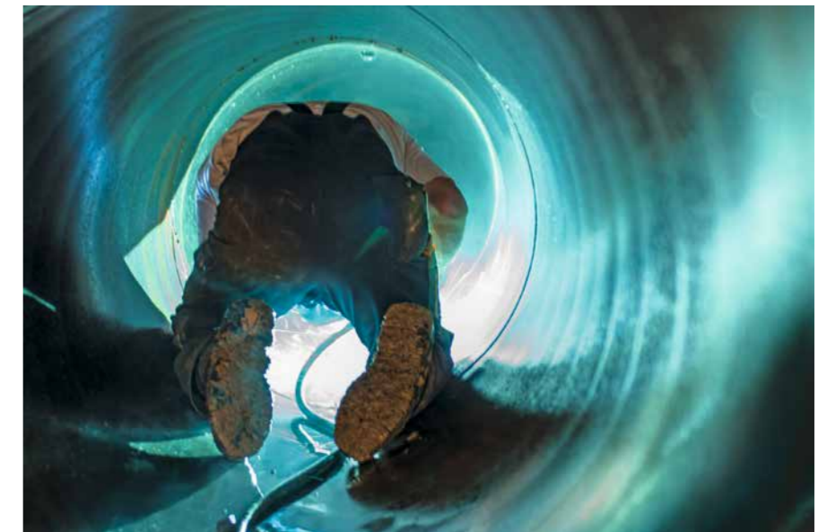
Installation of steel pipes for the district heating system. ▶
