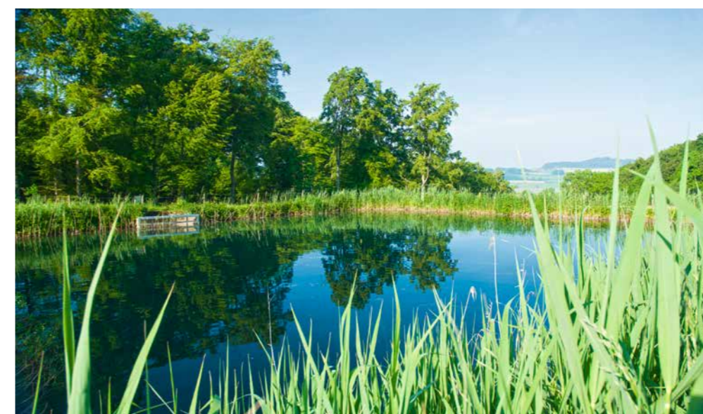
◀ In Wellnau, above Triengen, surface water is stored in TRISA's own reservoir.
